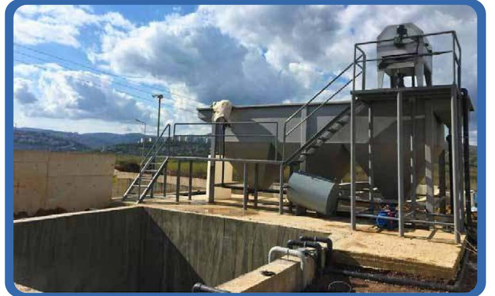
**GDF – Open dissolved air flotation units for handling high sludge loadings**
